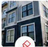
Exterior Paint & Repairs
